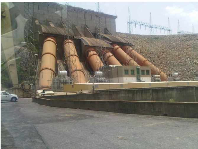
Above: the six penstocks (before ZINGA application) Right: 450 ton crane.
